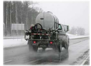
VDOT applying liquid deicer (brine) during a snow storm. Photo courtesy of VDOT
