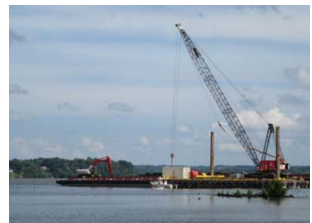
Work barge crews install marine mattresses. Photo by Glenda Booth
