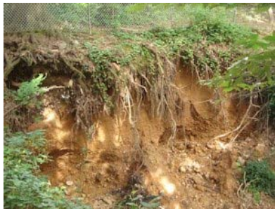
Severe streambank erosion in Mount Vernon Park sends sediment into Dyke Marsh during storms. Photo by Glenda Booth
