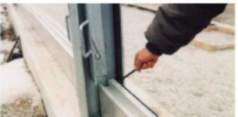
BASE ALUMINUM PLANK GASKETS SET DRY SIDE. THE PLANKS FILL WITH WATER AS FLOOD HEIGHT INCREASES, CREATING AREA STABILITY AND INTEGRITY. THE SEAL ON THE PLANK AND VERTICAL SURFACE FORMS THE "WET JOINT."
