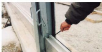
BASE ALUMINUM PLANK GREETS WET/DRY SOIL. THE PLANKS FILL WITH WATER AS FLOOD HEIGHT INCREASES, CREATING AREA STABILITY AND INTEGRITY. THE BEP ON THE PLANK AND VERTICAL SUPPORT FORMS THE "WET SOIL".
