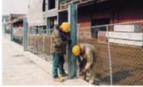
THE DCW™ WALL INSTALLATION HAS EASY DISASSEMBLED COMPONENTS. VERTICAL PLATING BEP PILES ARE PLACED EVERY 10 FEET APART, THEN TWO ANCHOR BARS CONNECT EACH BEP PILE TO THE PLATE FOUNDATION.
