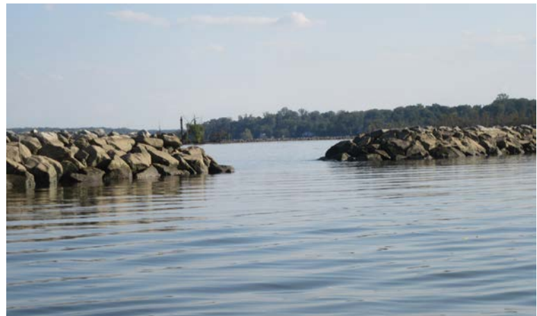
Rock sills built as part of the marsh stabilization project Photo by Glenda Booth
