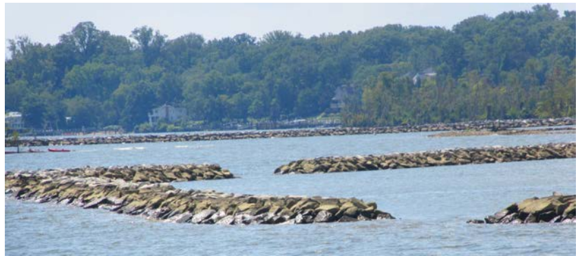
The Corps of Engineers built a breakwater (in the distance) to replicate a former promontory and five stone sills (foreground) for further protection.
